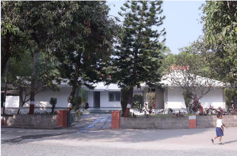
Renovated Ulhas playground | Kalyani Shala Balamandir and primary section
